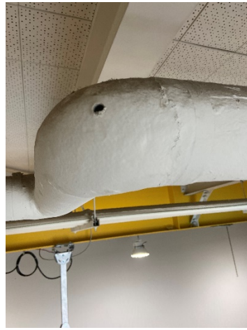
Example of the asbestos containing 6" OD Hardpack Pipe Elbow Insulation.
