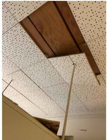
View of the nailed-on ceiling tiles.
