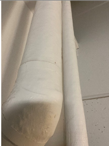
Example of the asbestos containing 8" OD Hardpack Pipe Elbow Insulation.
