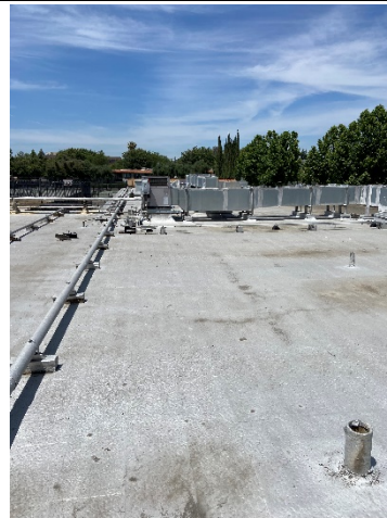
Example of the painted composition asphalt rolled roofing.
