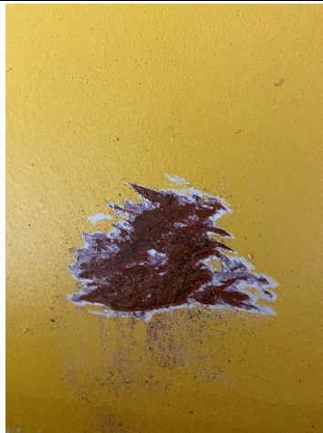
Example of the Yellow Colored Lead-Based Paint on the structural I-Beams located inside the Gym Buildings.
