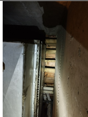
Example of the 6" OD Hardpack Pipe Insulation above the HVAC Duct. The insulation around these pipes are assumed asbestos containing materials.
